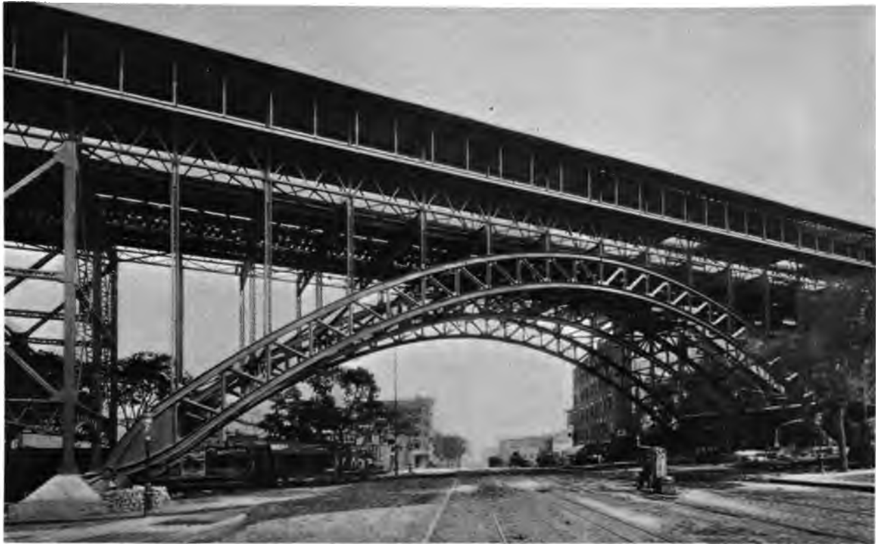
COMPLETED ARCH AT MANHATTAN STREET
